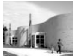
Citation Entry name Educare Name RDG Planning and Design Firm RDG Planning and Design Owner(s) Susan A. Buffet Foundation / OPS City Omaha, NE Photographer(s) Farshid Assassi Contractor Kiewit Construction Company
