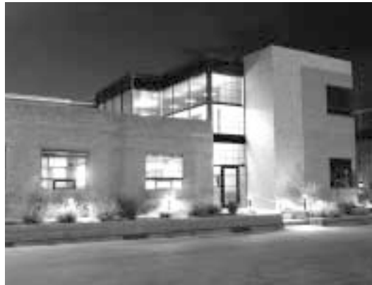
Honor Entry name Hughes Brothers Office Addition Name Cristy Pickrel, AIA Firm studioNRG, LLC Owner(s) Hughes Brothers City Seward, NE Photographer(s) studioNRG, LLC Contractor Ayars & Ayars, Inc.
